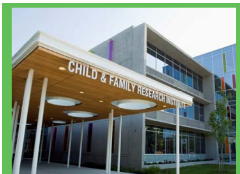
CUPIC facilities will occupy the fifth and fourth floors of the new Translational Research Building, pictured here. The building is located at the BC Children's Hospital in Vancouver, BC.
